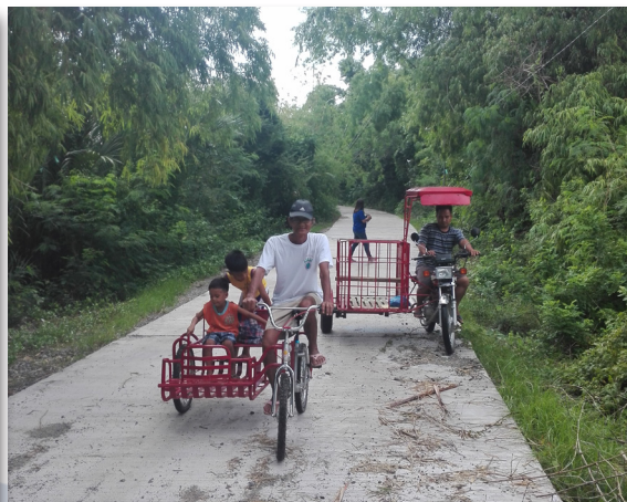
Concreting of Farm-to-Market Road Lingayen, Pangasinan
