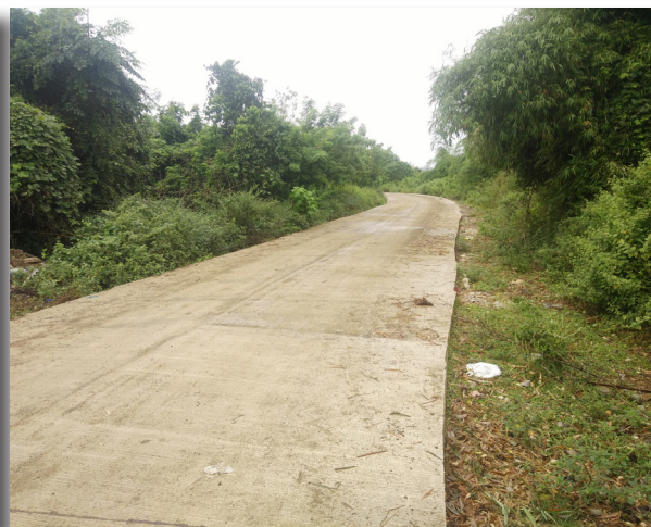
Upgrading of Farm-to-Market/Access Road Batac City, Ilocos Norte
