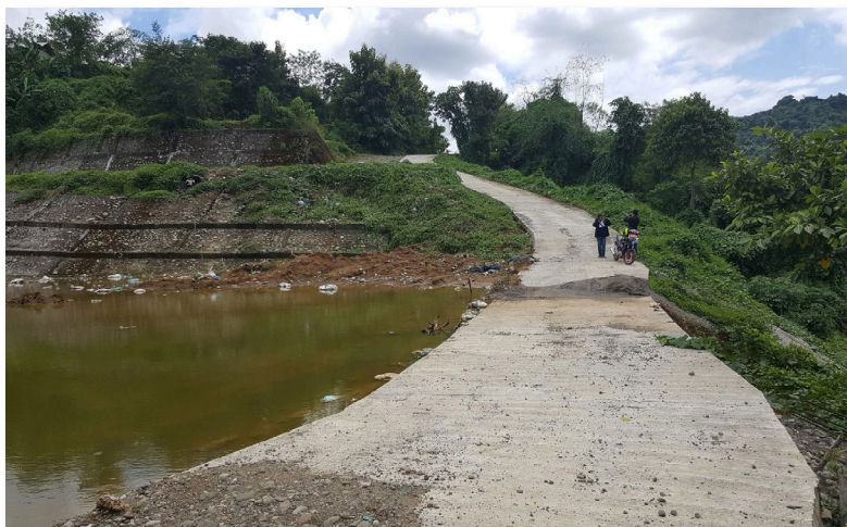
Upgrading of Dumpsite, Tubao, La Union
